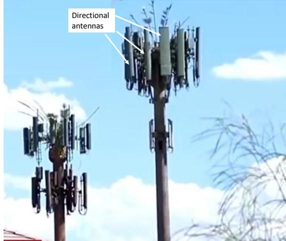
**Figure 1.** Directional antenna units are pointed at various directions around the pole to provide radial coverage in a specified living area.
